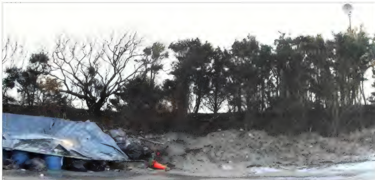
Figure 5.120. View looking southeast at Missile Maintenance Area historic earthwork, NIKE launch site. In addition to the recycling containers visible on the left, a debris pile from the state's beach cleaning program sits at the toe of the earthwork. The debris obscures the highly engineered shape of the earthwork and should be carefully removed to avoid damaging this feature (Olmsted Center, January 2009).
